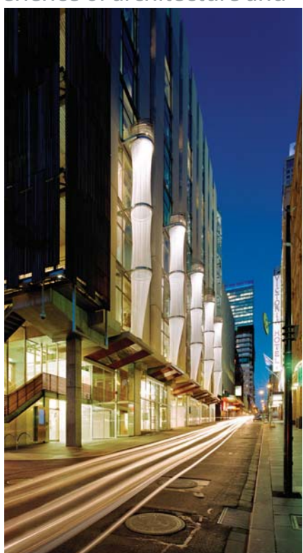
CH2 demonstrates regenerative principles where "shower towers" cool for free.
